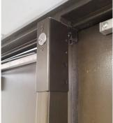
Remove the key from the mechanism and set the Mullion safely aside in a location where it will not fall onto anyone or anything. Return Key Ring #25 to CMO.
